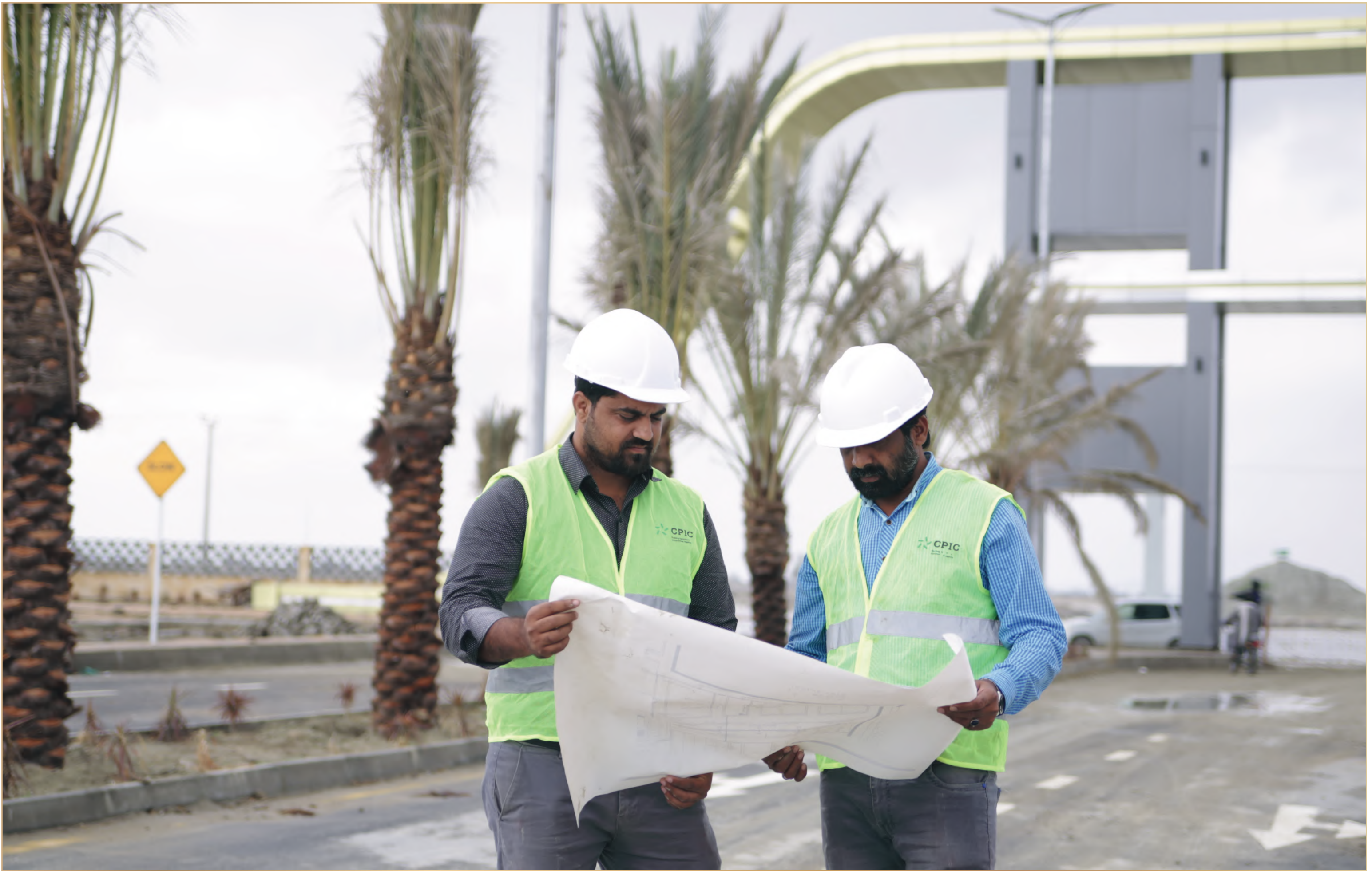
International Port City construction in progress
