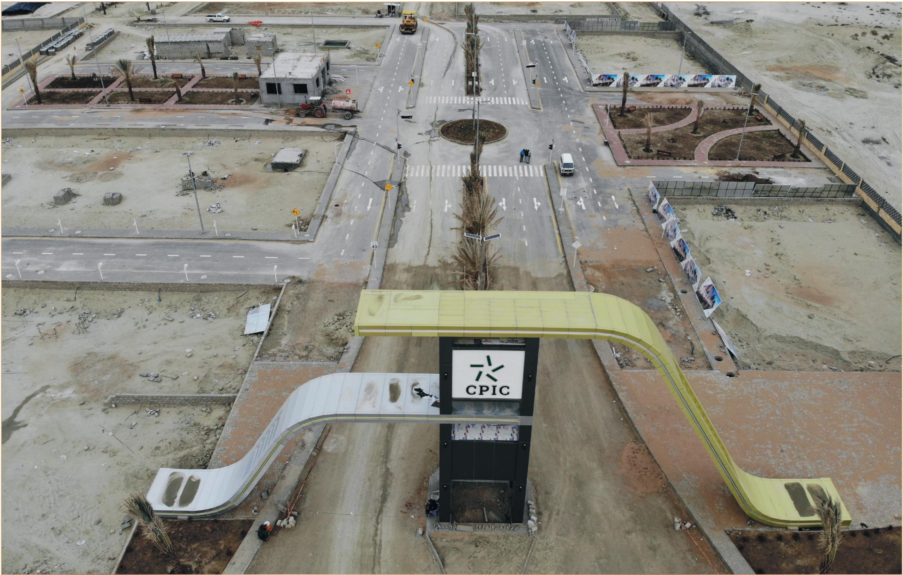
Drone shots of International Port City construction site
