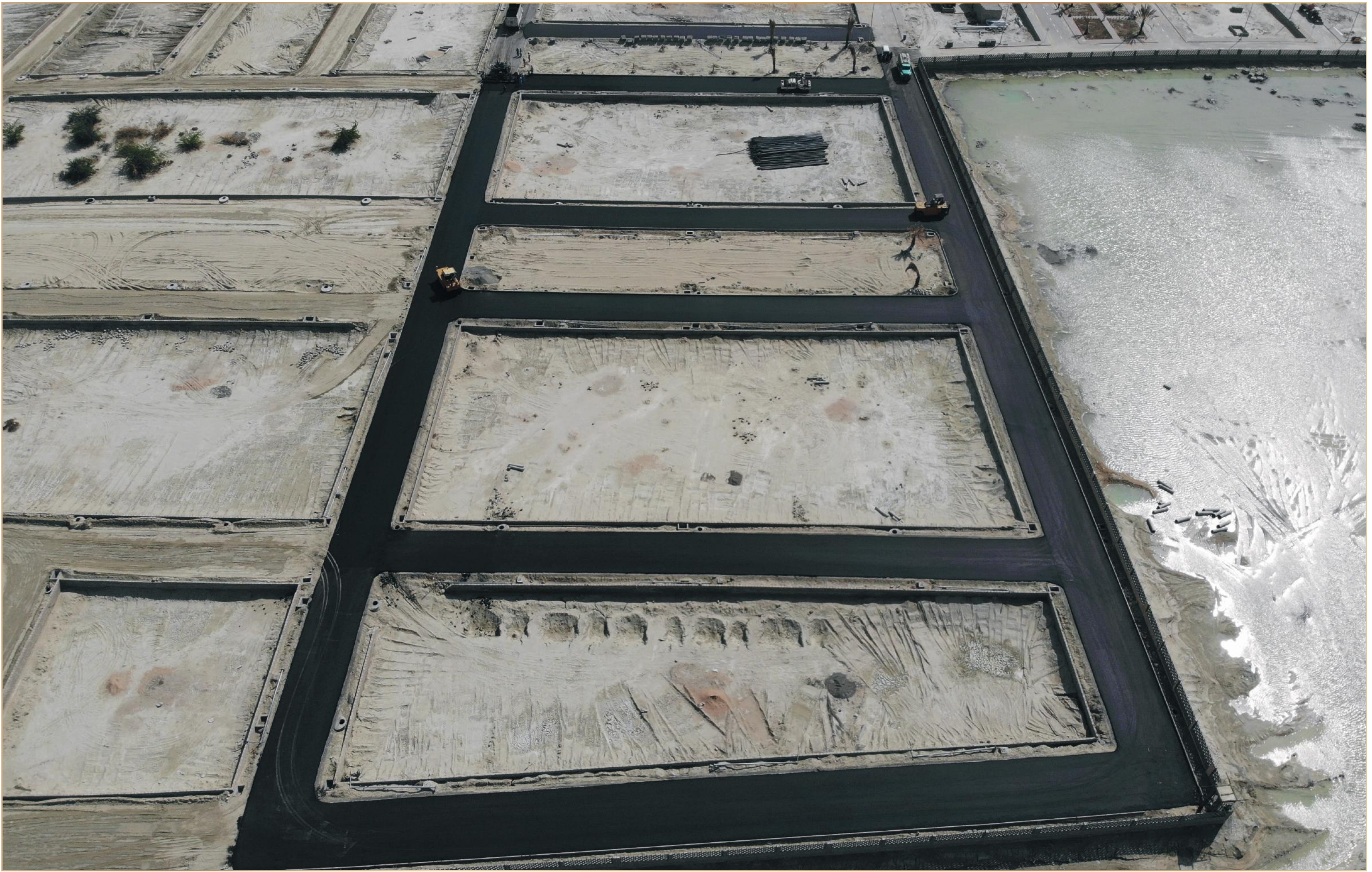
Construction of roads in Zone B at International Port City site
