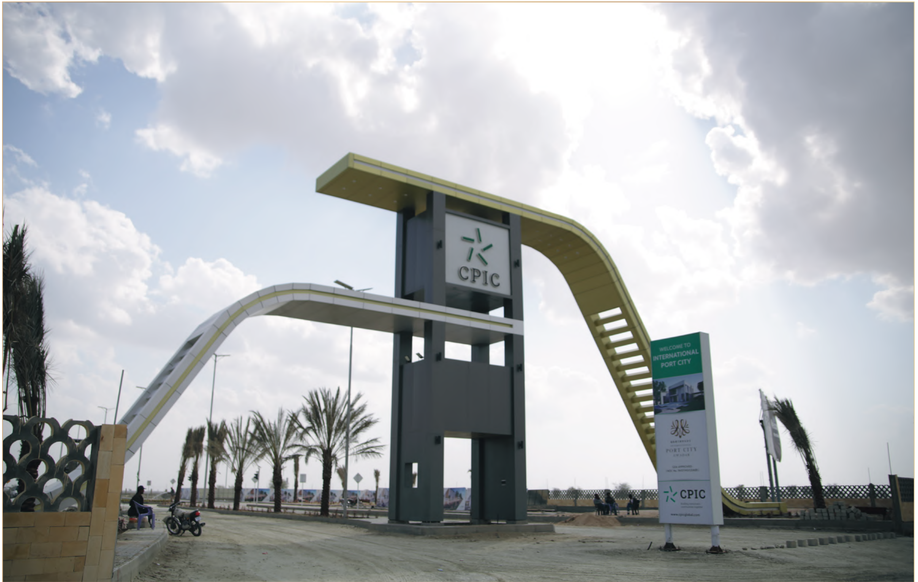
Main Gate views at International Port City
